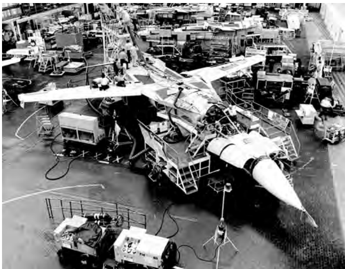
F-111As were modified to the EF-111A configuration by Grumman Aerospace Corporation at its Riverhead Plant, Long Island, NY. The photo shows several F-111As in various modification stages. (Courtesy of Northrop Grumman Corporation)
